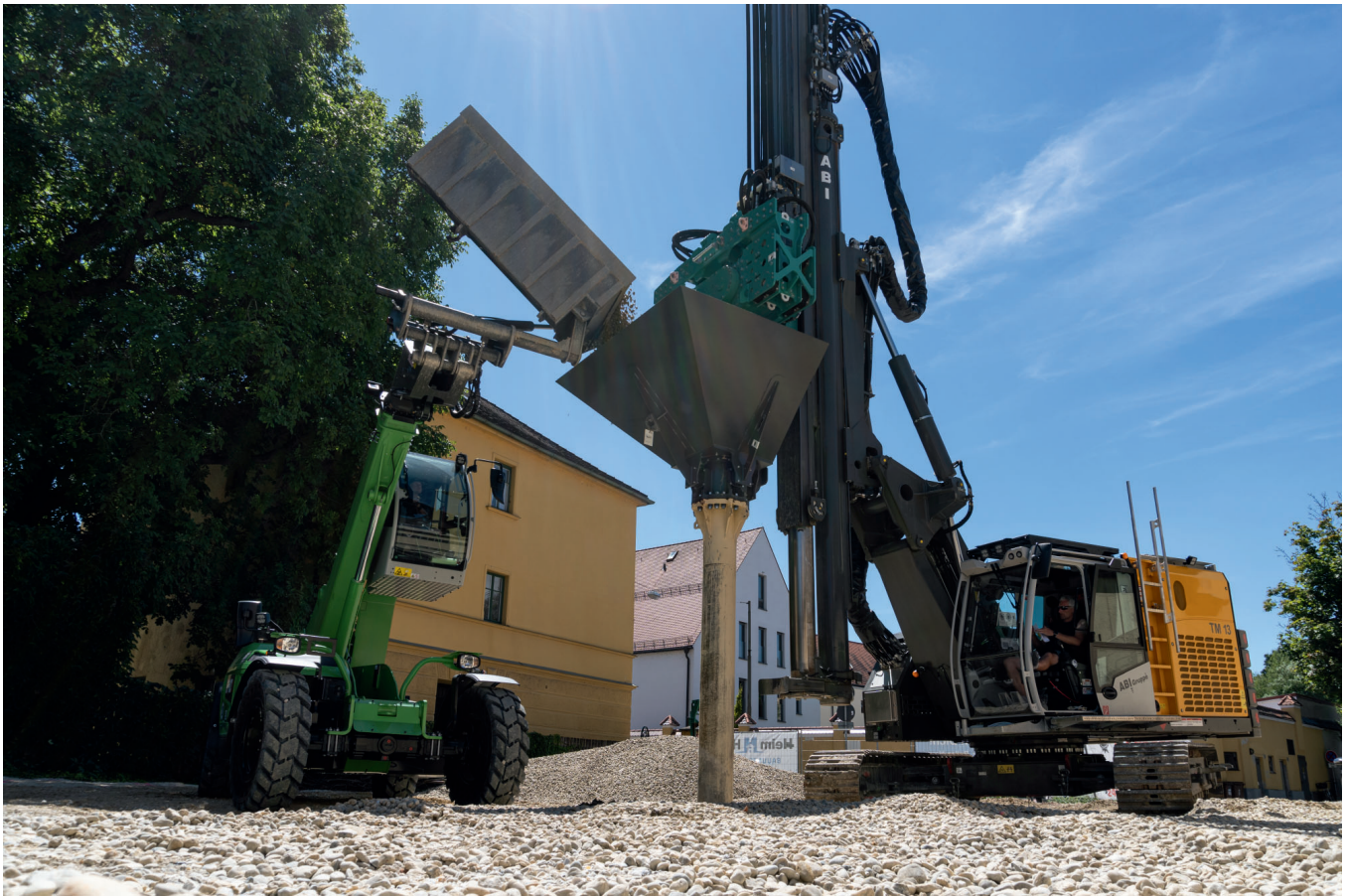
Photo: The hopper is filled with gravel bevor extracting the probe
