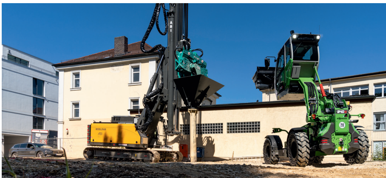
Photo: Installation of stone columns for soil improvement
