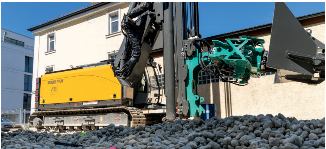
Photo: Set-up - the guiding carriage with hinged joint is mounted on leader mast
