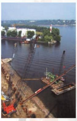
HPH6500 on European swinging leads driving HP400 x 47m long on 1.4:1 rake (approx. 32º to the horizontal) – Hamburg, Germany
