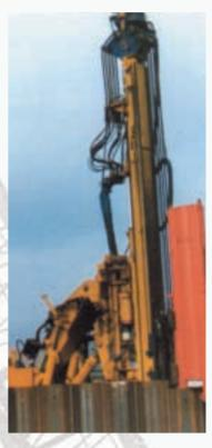
HPH1200 on ABI Mobilram driving pairs/single steel sheet piles - UK
