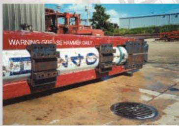
HPH2400 fitted in 26" American leads driving 12" H-pile on a 2:3 batter – Chicago, IL, USA Note the simple lead guide design with H-pile guide box fitted in place of standard Leg Inserts
