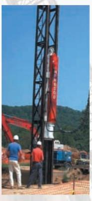
HPH6500 on 32" American leads driving 14" H-pile x 130' long to bearing of 450 ton – Northern Kentucky, USA
