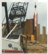
HPH1200 running from H&M Vibrator Power Pack - USA
