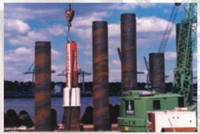
HPH6500 with Ø1420 Guide Sleeve driving 30m long Combi-Wall Caissons – Hamburg, Germany
