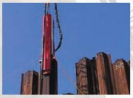
The addition of a simple spreader plate under the standard drive cap or Anvil permits all Dawson hammers to achieve almost total head coverage on any pair of sheet piles. This significantly reduces the likelihood of pile top damage in difficult driving.
