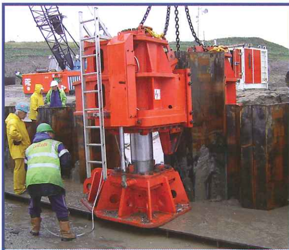
X1000t Universal Pile Extractor pulling Arcelor AZ36 sheet piles – Easington, England
