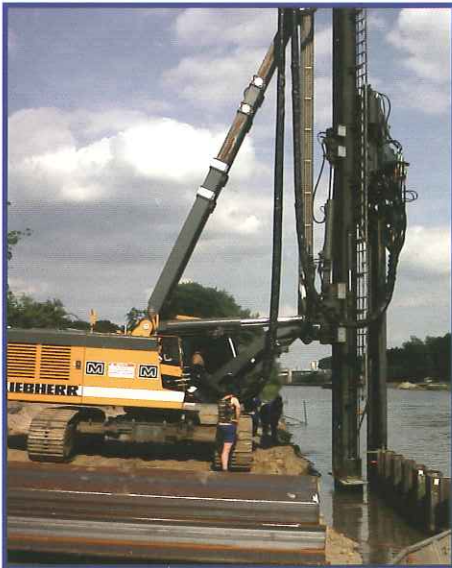
2 Cylinder Push-Pull on Liebherr LRB 155 piling rig installing U & Z-piles - Germany
