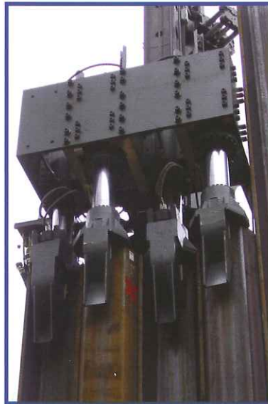
4 Cylinder Push-Pull on Liebherr LRB 255 piling rig installing U-piles - UK
