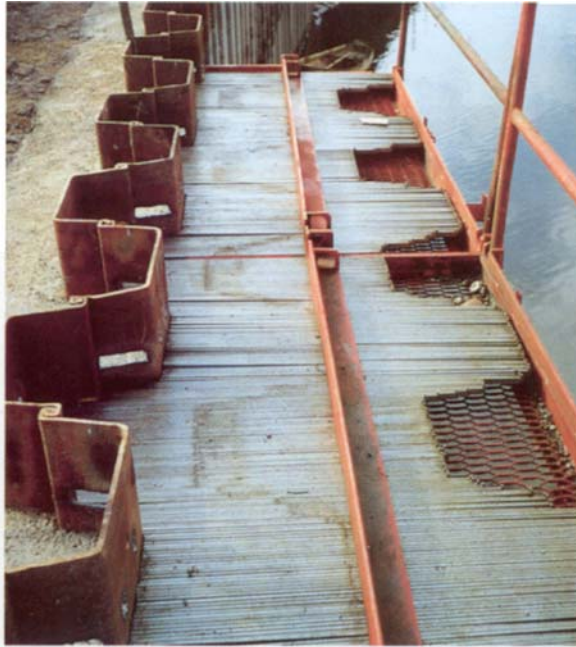
(left) Pile capping at Whitstable Harbour, Kent, shows clearly soffit panels following the shape of Larsen profiles. Main Contractor: John Shelbourne Ltd. (Costain)
