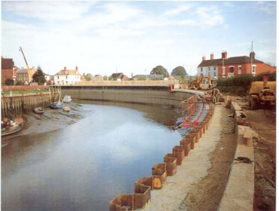
(left) Pile capping at Whitstable Harbour, Kent, shows clearly soffit panels following the shape of Larsen profiles. Main Contractor: John Shelbourne Ltd. (Costain)
