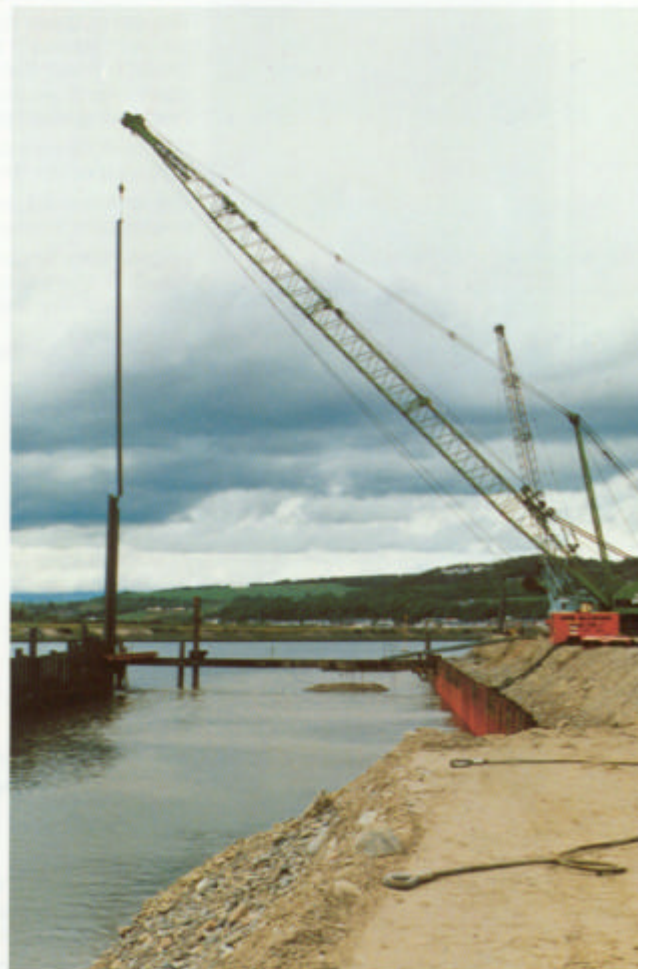
(left) Attaching the Pile Threader during a piling operation at Namur on the River Meuse in Southern Belgium. (right) Construction of a new quay at Inverness, Scotland. 1600 tonnes of Larsen 6 sheet piling were driven with the aid of the Pile Threader.
