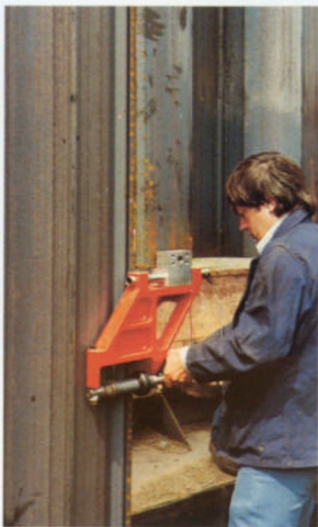
(left) Attaching the Pile Threader during a piling operation at Namur on the River Meuse in Southern Belgium. (right) Construction of a new quay at Inverness, Scotland. 1600 tonnes of Larsen 6 sheet piling were driven with the aid of the Pile Threader.
