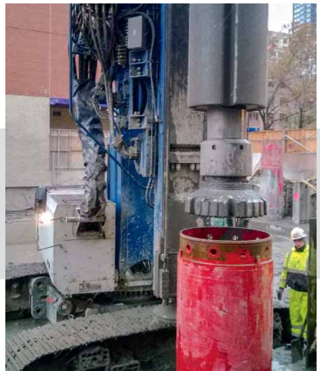
DELMAG drill rig using a down the hole hammer in hard, rocky ground.
