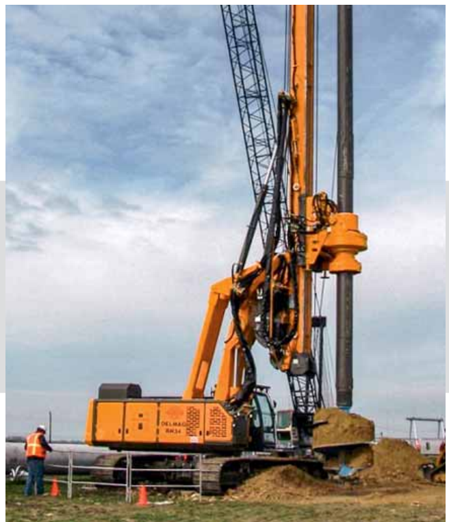
Uncased Kelly drilling with a short leader mast foot: The short leader mast foot enables larger diameters to be drilled, as the drilling tool can rotate underneath the leader mast.
