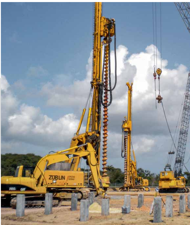
Manufacture of drilled-in-situ concrete piles. The achievable depth can be extended using a concrete Kelly extension.
