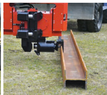
Handling of H beam
