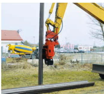
Positioning, aligning, and driving
