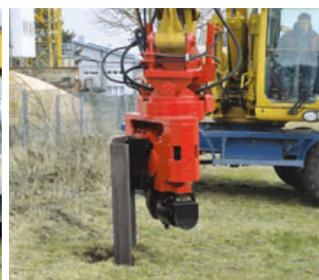
Shifting and driving to final depth
