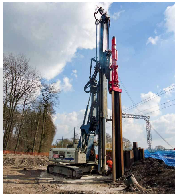
Driving steel sheet piles. DELMAG diesel pile hammer is often used for back driving or for embedding piles in a load bearing layer.
