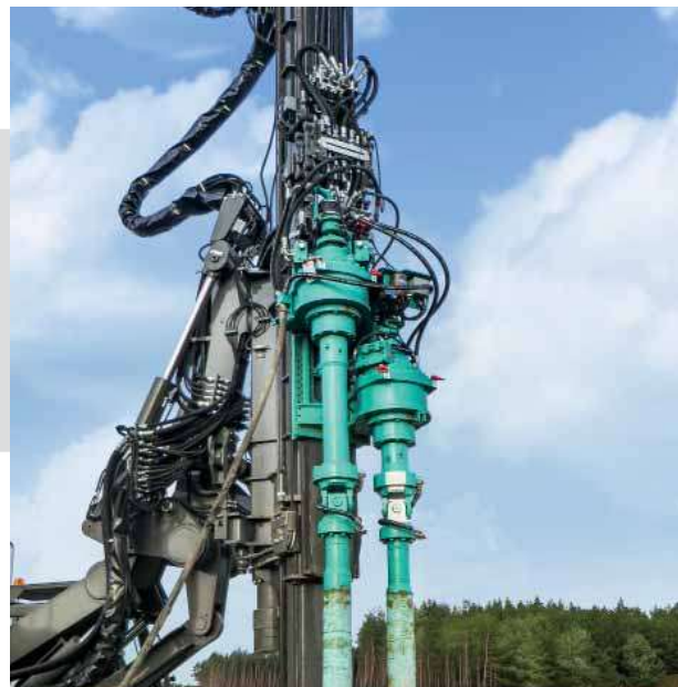
For soil mixing, productivity can be increased by using multiple auger drives.
