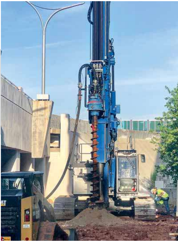
Installation of continuous flight auger piles: after reaching the desired depth during extraction concrete is pumped through the hollow stem of the auger.
