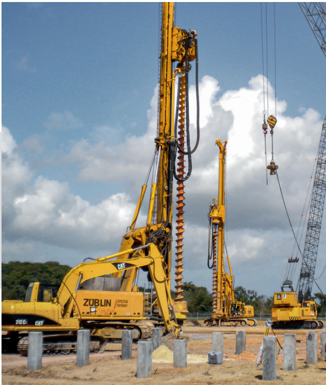
Manufacture of drilled-in-situ concrete piles. The achievable depth can be extended using a concrete Kelly extension.
