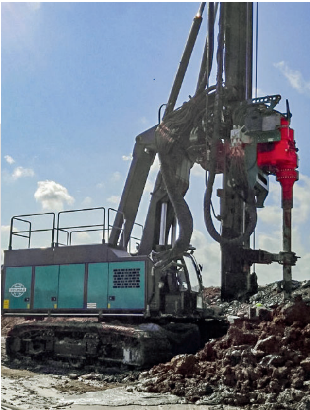
Soil mixing (WSM) using an RHP 150 auger drive to increase the load-bearing capacity of the soil. The existing soil material is mixed with a suspension additive.
