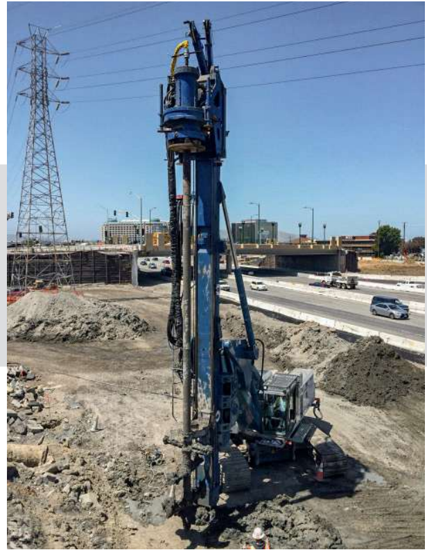
Drill rig in a short leader mast application with limited headroom: The required depth is achieved by installing additional pipe sections on the mixing rod.
